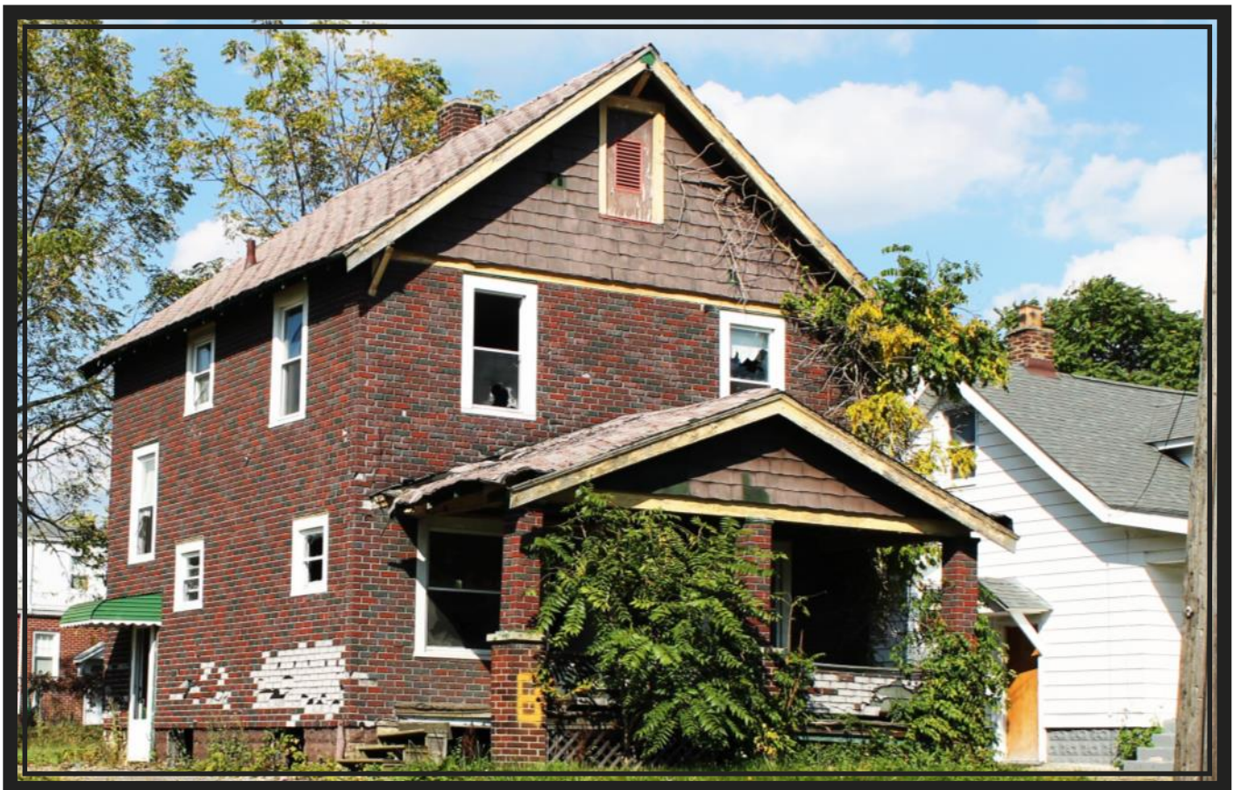
A vacant, unsecured home sits just one block from Taft Elementary School.
